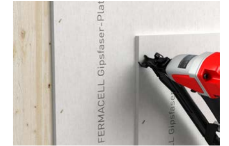
Fixing board in board.
