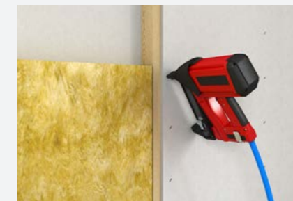
Stapling to timber substructure
