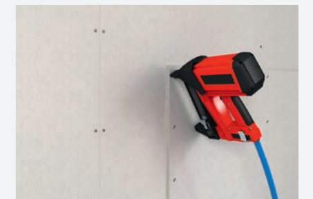
Stapling fermacell® fibre gypsum board to fermacell® fibre gypsum board
