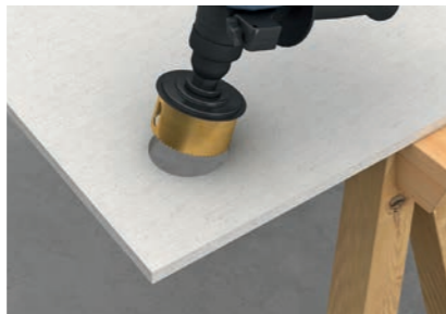
Milling out socket holes
