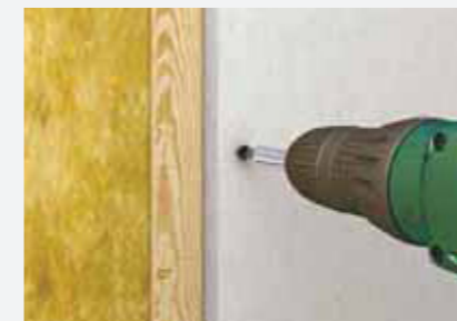
Screwing to timber substructure
